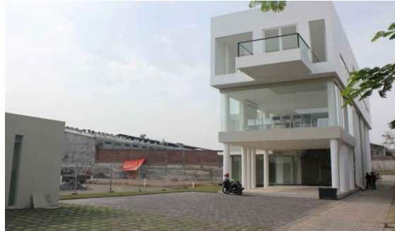
GRAHA NATURA KANTOR PROJECT / SITE OFFICE
